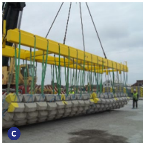
A Offshore Support Vessel EDT Protea DP III B Seaeye Panther Plus 920 C Mattress installation frame D 3D impression of A15 and B10 platforms, pipelines and umbilicals E Diving lars
